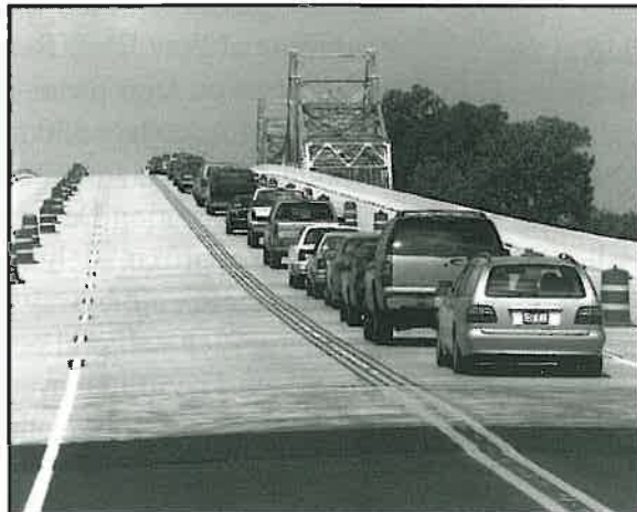
Cars cross the new Augusta Bridge after the dedication. The old steel-structured bridge can be seen in the background.
