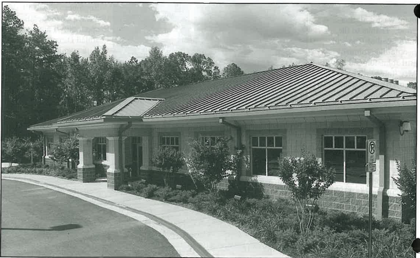
Front view of the administrative office of the Materials testing facility
